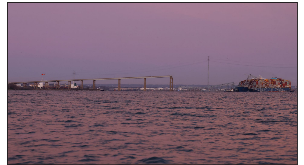
A view of the Dali cargo vessel after it crashed into the Francis Scott Key Bridge, causing it to collapse in Baltimore, MD.
